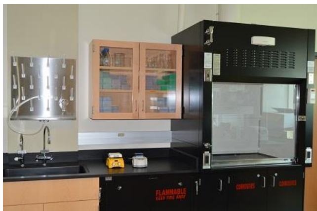
Picture of Mott fume hood next to sink.
