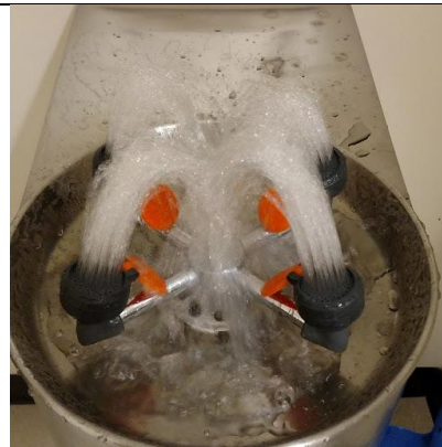
Picture of an activated eyewash.
