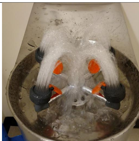
Picture of an activated eyewash.
